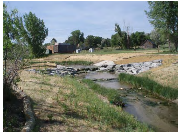
Photo 9 – Constructed Channel & Grouted Boulder Drop Structure
