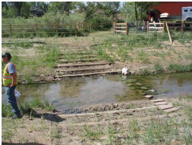
Photo 10 – Constructed Channel & Equestrian Crossing
